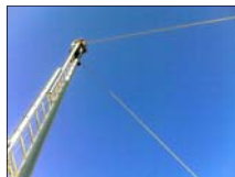
Engineer Soule reaches the top of the pole.
