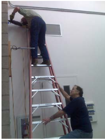
Jack Kuhn and Dave Goelz prepare for curtain installation.
